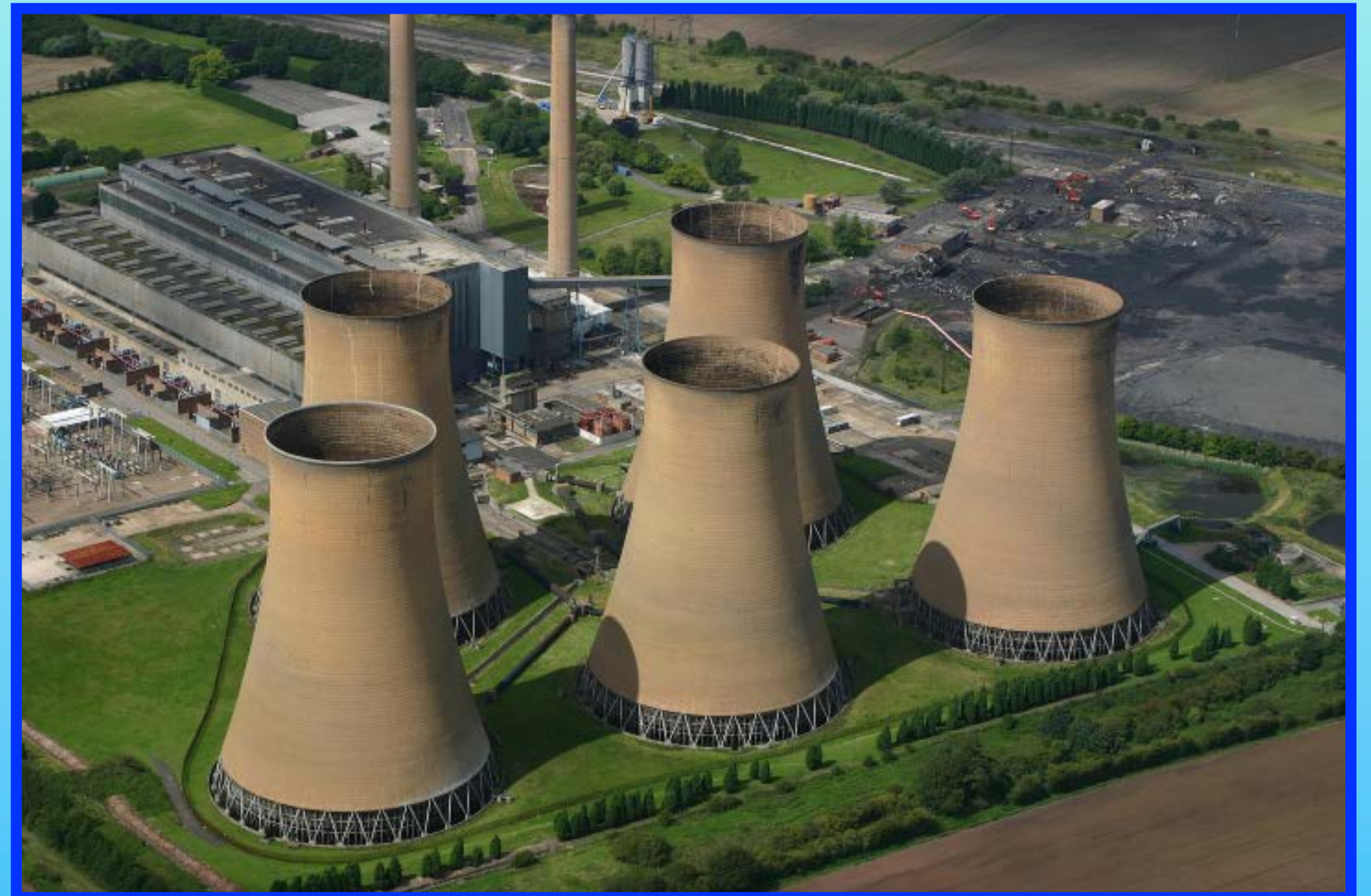
Ratcliffe-on-Soar Power Station, Nottinghamshire
